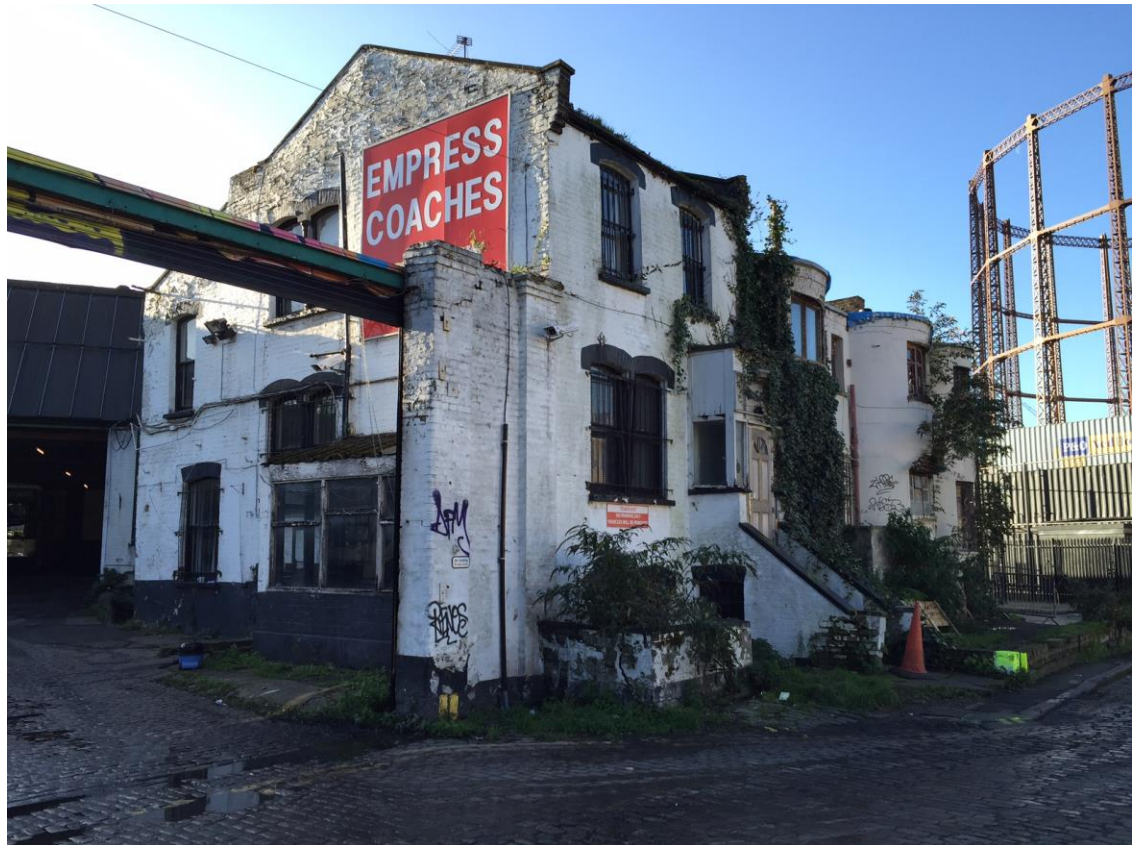
Figure 5 (above): View of the existing historic cottages on site to be refurbished
