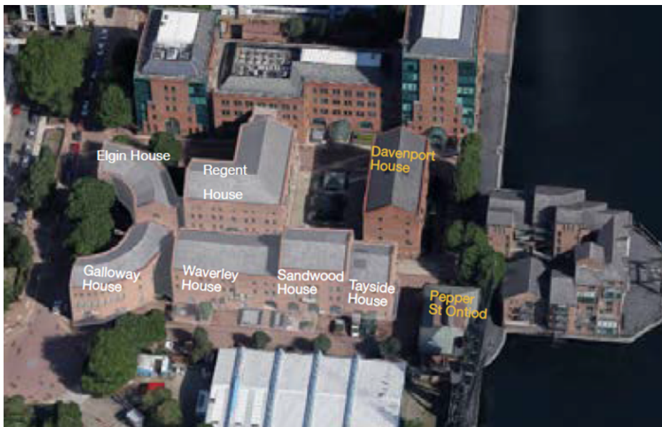
Fig.2 – Aerial View of Application Site
